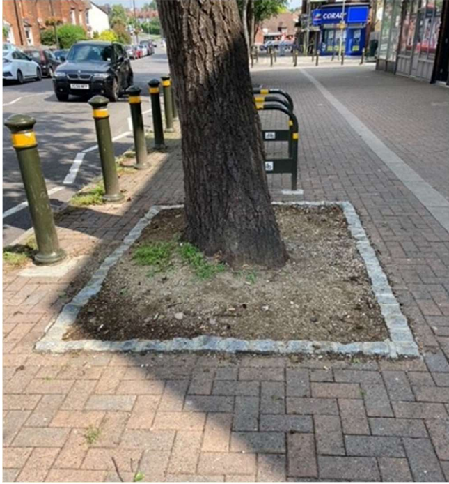
Tree base repair work, enlarged tree pits edged with granite setts
