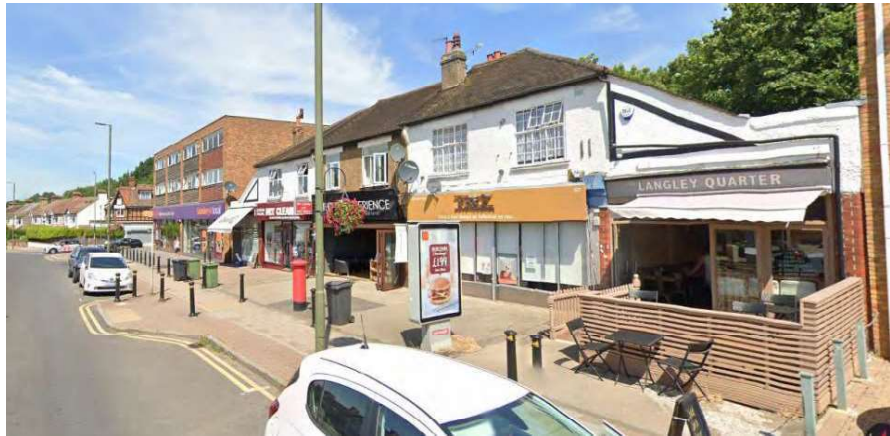
Lamp column repainting, pavement resurfacing
